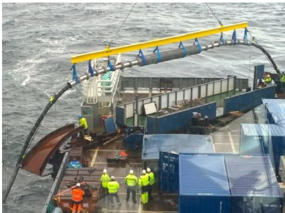
Figure 43 : Joints de câble
