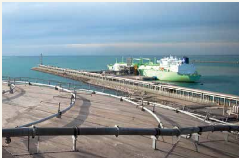
◀ LNG carrier at the terminal in Fos Cavaou.
